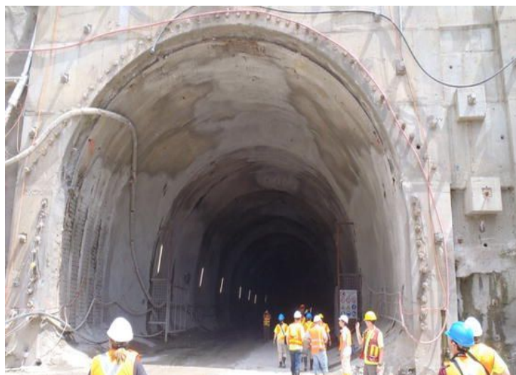
Figure 2.1: Tunnel San Fedele, Switzerland (tunnelingonline, 2019)
