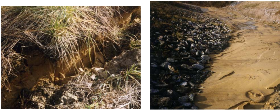
(a) Cracks widening between sliding blocks (b) Vegetative support soils washed to slope base
